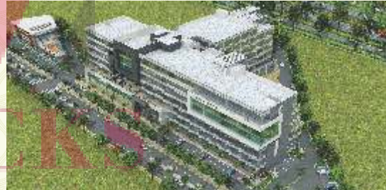
Success Tower, Sector-65, Gurgaon
